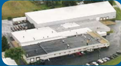
Mitek Facility: Monroe, Wisconsin
