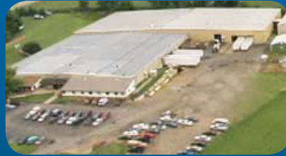
Mitek Facility: Winslow, Illinois
